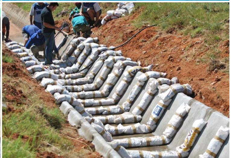
Sand bags can be used to compress joints during setting
