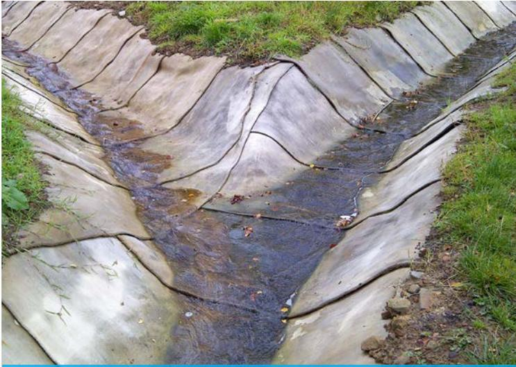
CC can be easily manipulated to form ditch junctions and terminals
