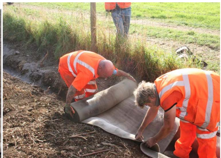
CC being laid using batched rolls
