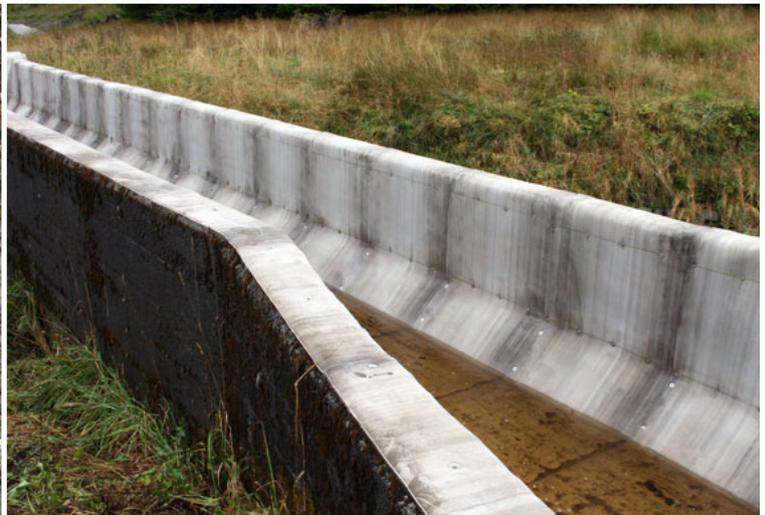
CC can also be used to reline existing concrete water channels
