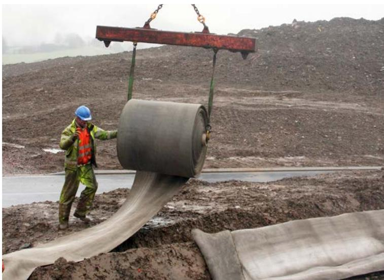
CC bulk roll being laid using a spreader beam
