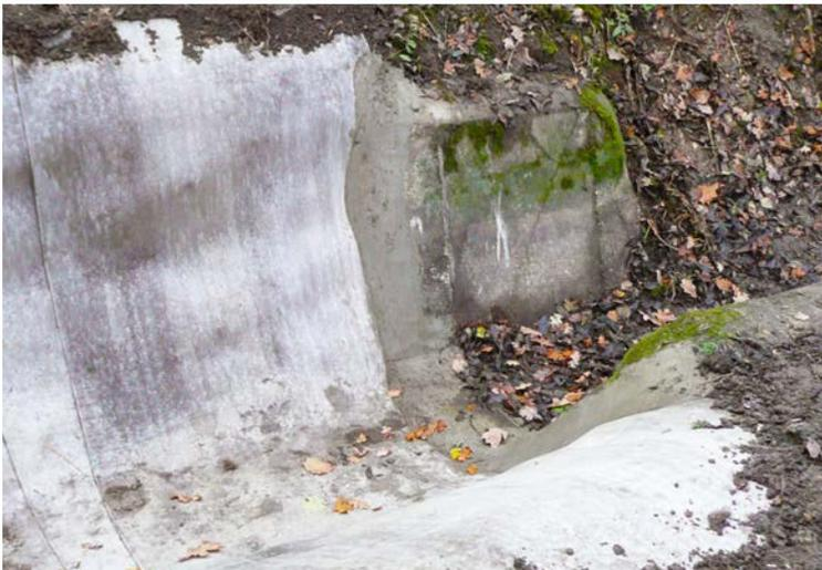
A suitable mortar can be used to join and seal CC to existing infrastructure
