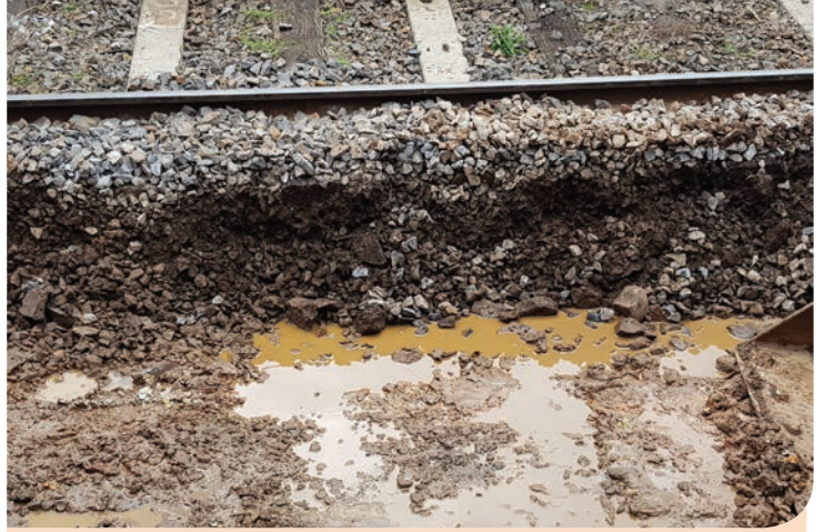
Susceptible mud-pumping formation.
