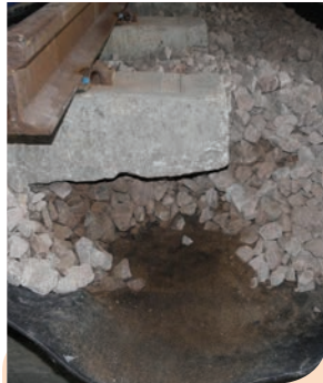
Successful pumping test using Tracktex.
