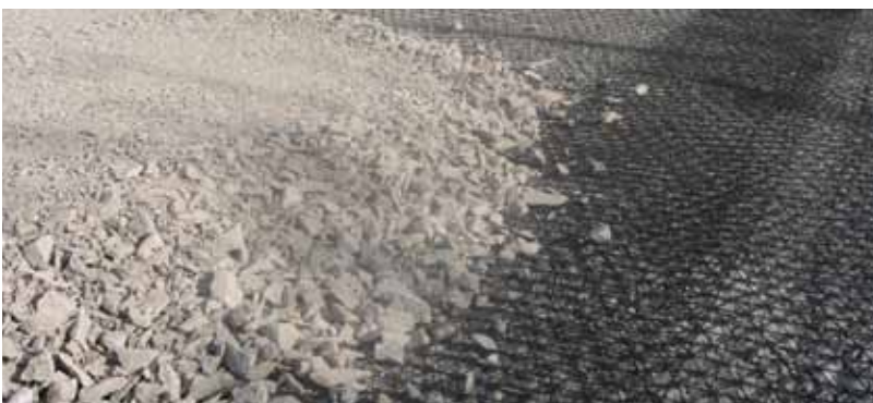
Improving and strengthening the A66 in Melsonby
