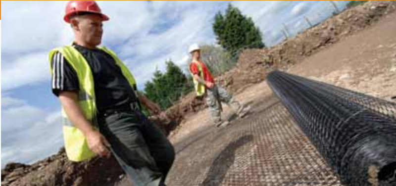
TriAx installation, Stoke
