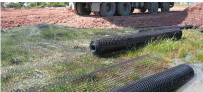
Stabilising ground to facilitate off-road parking at Lanarkshire
