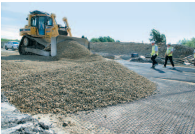
Using Tensor TriAx Geogrids reduces up-front costs and future maintenance.
