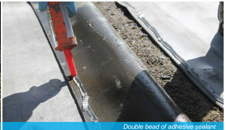
Double bead of adhesive sealant
