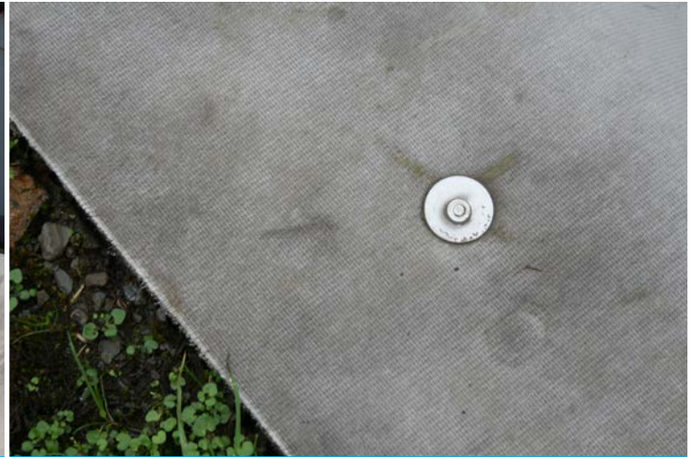
CC anchored using a fired concrete nail with a 20mm washer
