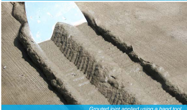
Grouted joint applied using a hand tool
