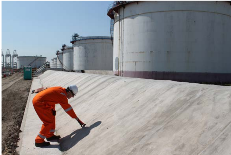
CC captured with a poured concrete curb
