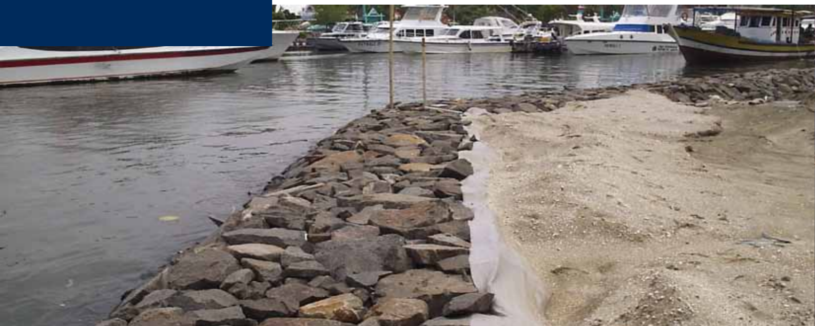
Rubble containment dyke with geotextile filter
