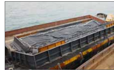
Geocontainer® offshore breakwater construction
