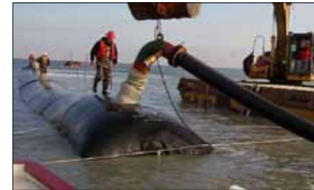
Geotube® containment dyke construction
