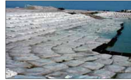
Geobag® revetment construction
