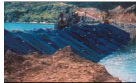
Mirafi® geotextile behind rock containment dyke
