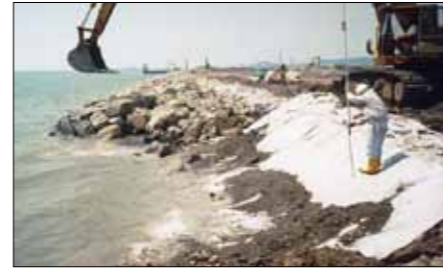
Polyfelt® geotextile beneath rock revetment
