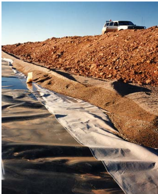
Decant causeway with Bidim geotextile protection layer over HDPE liner (A44)
