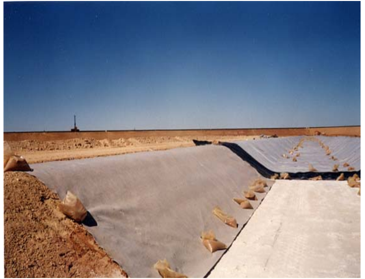
Decant drainage channel continued at a depth of 3 metres (gravity feed)
