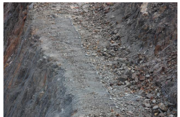
Anchors at the crest of one of the slopes
