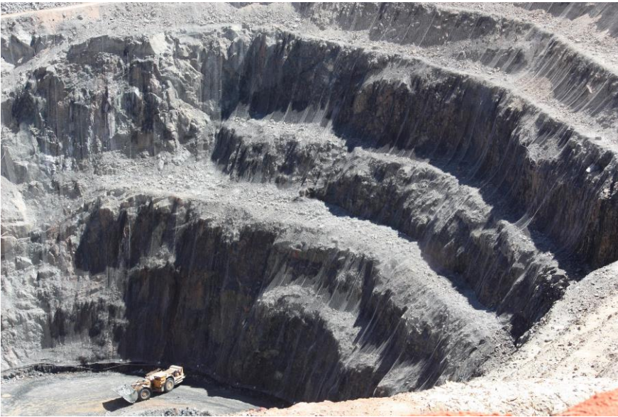
The Rockfall netting draped over five benches – roll lengths in excess of 120m long can be supplied if required
