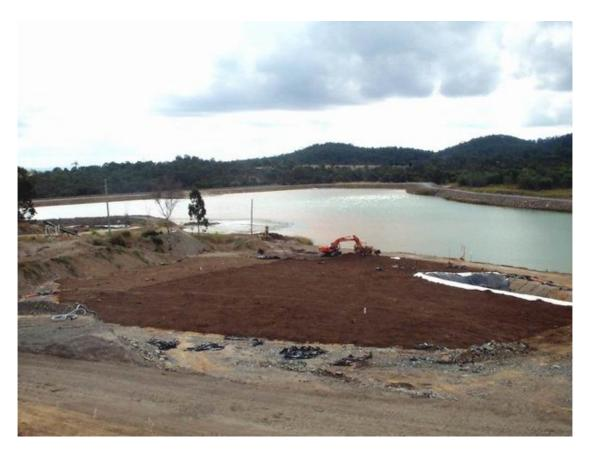
Photo 6 – Completed cell with leachate dam on RHS
