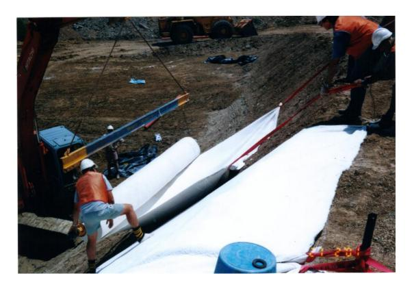
$\begin{array}{c} \textbf{Photo 1-Installation of ELCOSEAL \ GCL \ on \ the \ upstream \ tailings \ dam \ \\ \textbf{face} \end{array}$
