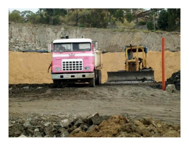
**Photo 5 – Filling of containment cell**
