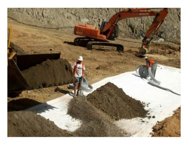
Photo 3 – Installation of Megaflo over-drainage on GCL
