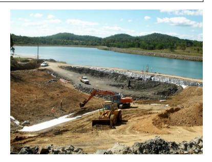
In order to recover precious metals from the flue dust material, an above-liner collection system was specified using a **Megaflo**<sup>®</sup> Flat Panel collection system.
