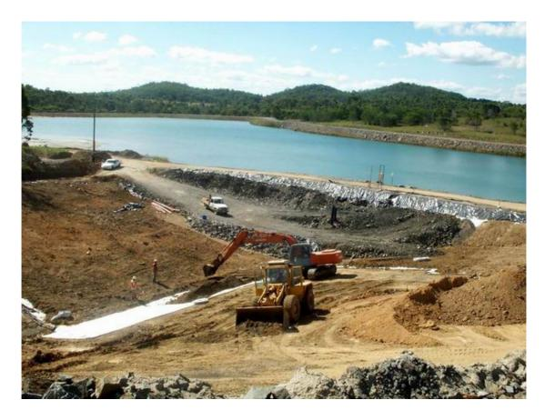
Photo 4 – Placement of waste rock & cover material
