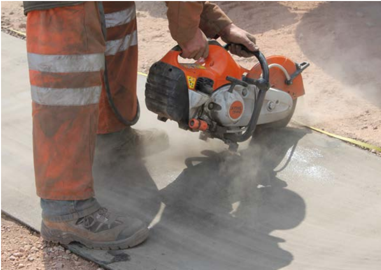
Unset CC8 cut to length using a disk cutter
