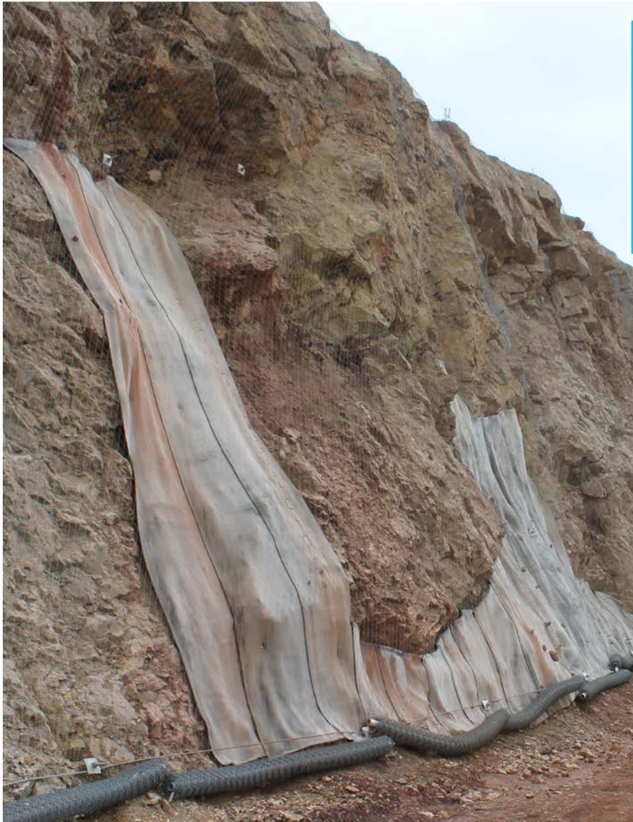
Post-set CC was draped in a wire mesh and the rock face stabilised using a thread bar system. Sections of slope were later blasted.
