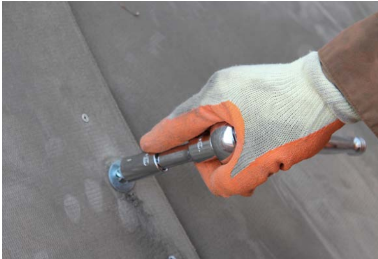
CC fixed to rock face at 2m intervals using 100mm rock bolts
