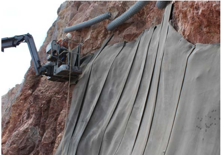
CC8 hung from top of rock face using 250mm steel ground pegs
