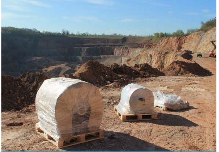
CC8 delivered to site in bulk rolls
