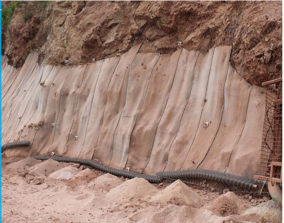
Completed section of slope lined with CC5
