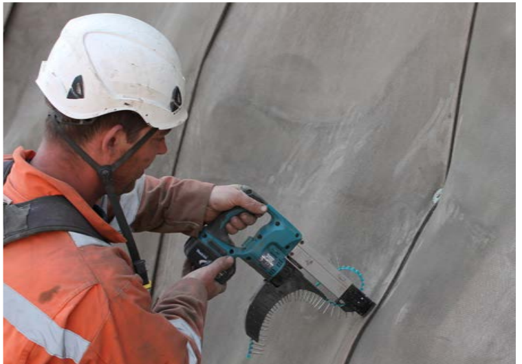
Adjacent lengths of CC fixed using autofeed screwdriver
