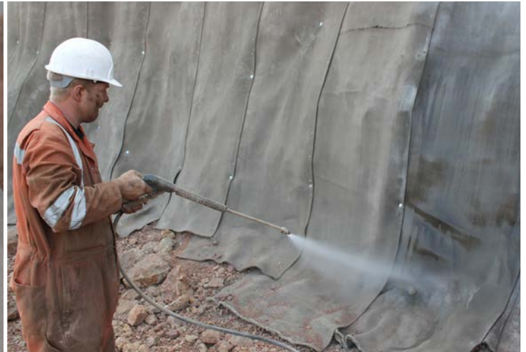
CC hydrated water from a 4000 gallon dust suppression tank
