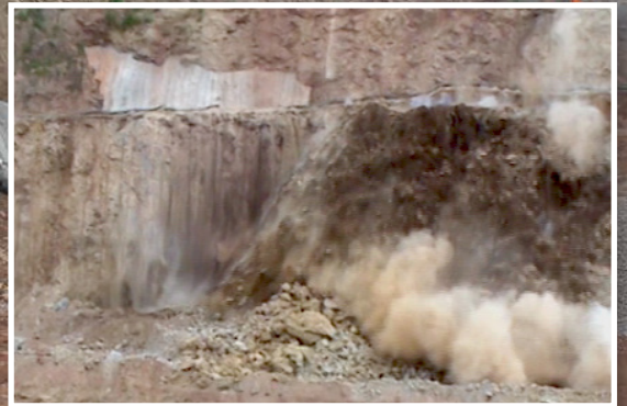
Post-set CC was draped in a wire mesh and the rock face stabilised using a thread bar system. Sections of slope were later blasted.
