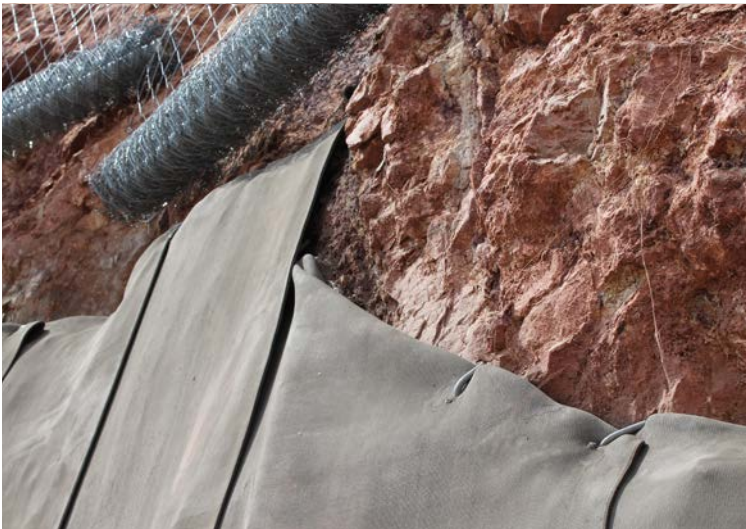
Adjacent lengths of CC overlapped by 100mm
