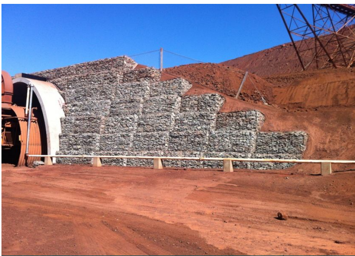
The Stepped Arrangement Of The Gabion Side Walls
