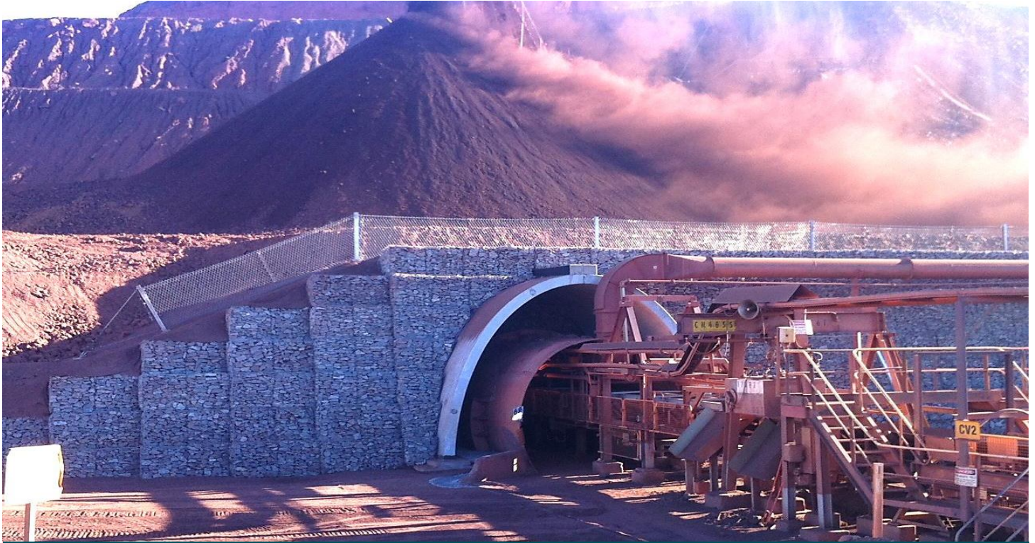
The Completed 7m High Mass Gravity Gabion North Wall
