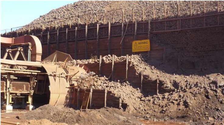
The Original Timber Sleeper North Wall
